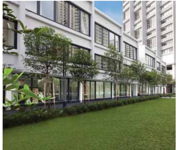
The Hub, Petaling Jaya , is adjacent to SDB's developments Five Stones and Ameera
